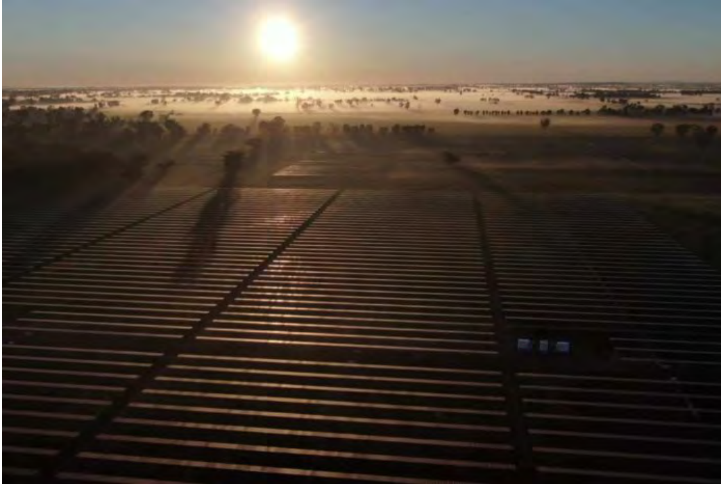
PHOTO: Sun rises over the Numurkah solar farm. (ABC News)
